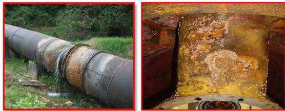
Figure 1: picture-showing corrosion in pipelines
